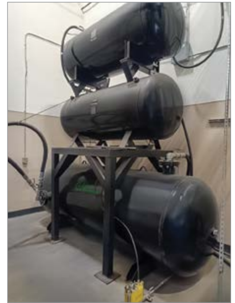
The tank system supporting the food processor’s modified atmosphere packaging for product freshness
